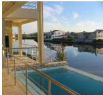
SIMPLE HORIZONTAL ELEMENTS IN STAINLESS STEEL
