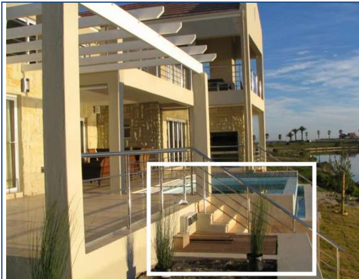
Pool pump & filters screened from view
